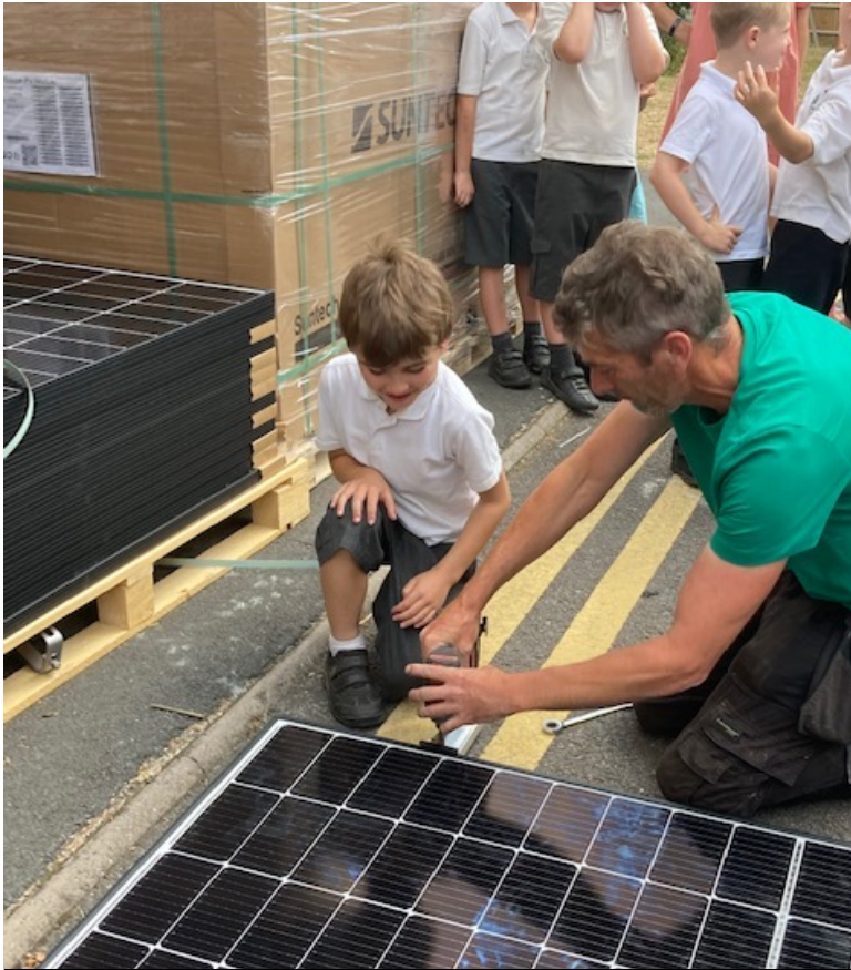
Ciaran one of the installers who works with the CBS, showing young students how a solar panel is fixed to a roof rail.
